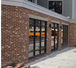
Examples of appropriate masonry walls
